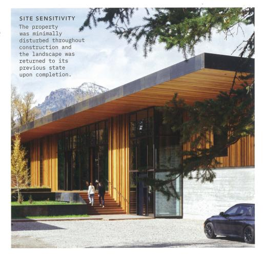
Cedar is also used for the soffit/ceiling system and the interior window trim. To enhance the wood's natural beauty, the cedar is finished with a clear stain. To specify nature's most versatile building material for these applications, the award-winning firm along with the homeowners opted for a premium clear grade.
