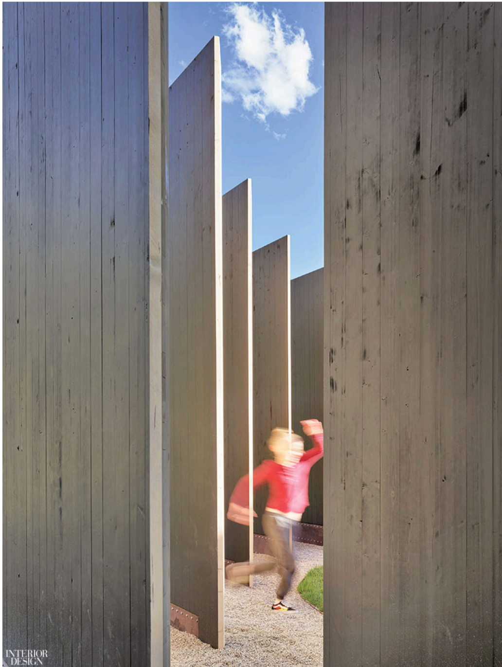
A steel foundation anchors 22 panels of graded spruce-pine-fir. Photography by Matthew Millman.
