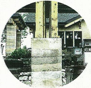
EARTHLY HOME Stephen Start's home on Lookout Mountain outside Spokane, Wash., has an outdoor pavilion with a colonnade of 16 rammed-earth columns made from 49 tons of compacted gravel. 'We wanted the house to feel almost like it came out of the ground,' said Mr. Start, above.
