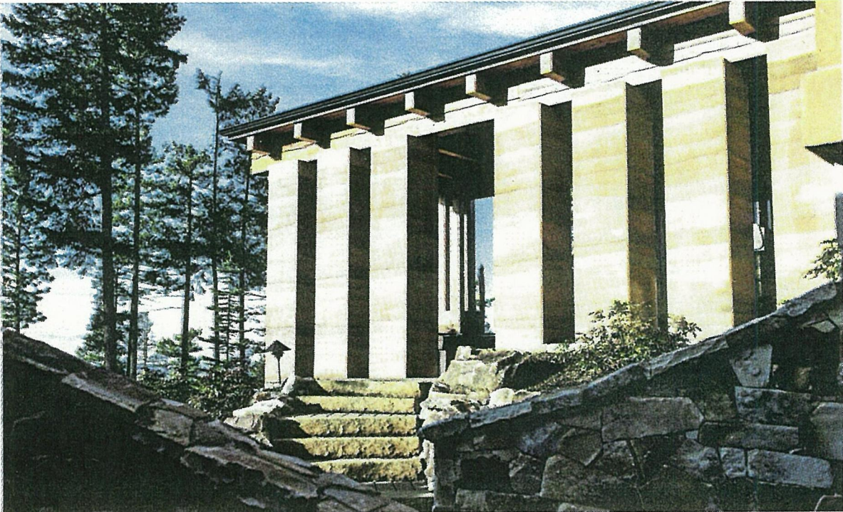
EARTHLY HOME Stephen Start's home on Lookout Mountain outside Spokane, Wash., has an outdoor pavilion with a colonnade of 16 rammed-earth columns made from 49 tons of compacted gravel. 'We wanted the house to feel almost like it came out of the ground,' said Mr. Start, above.
