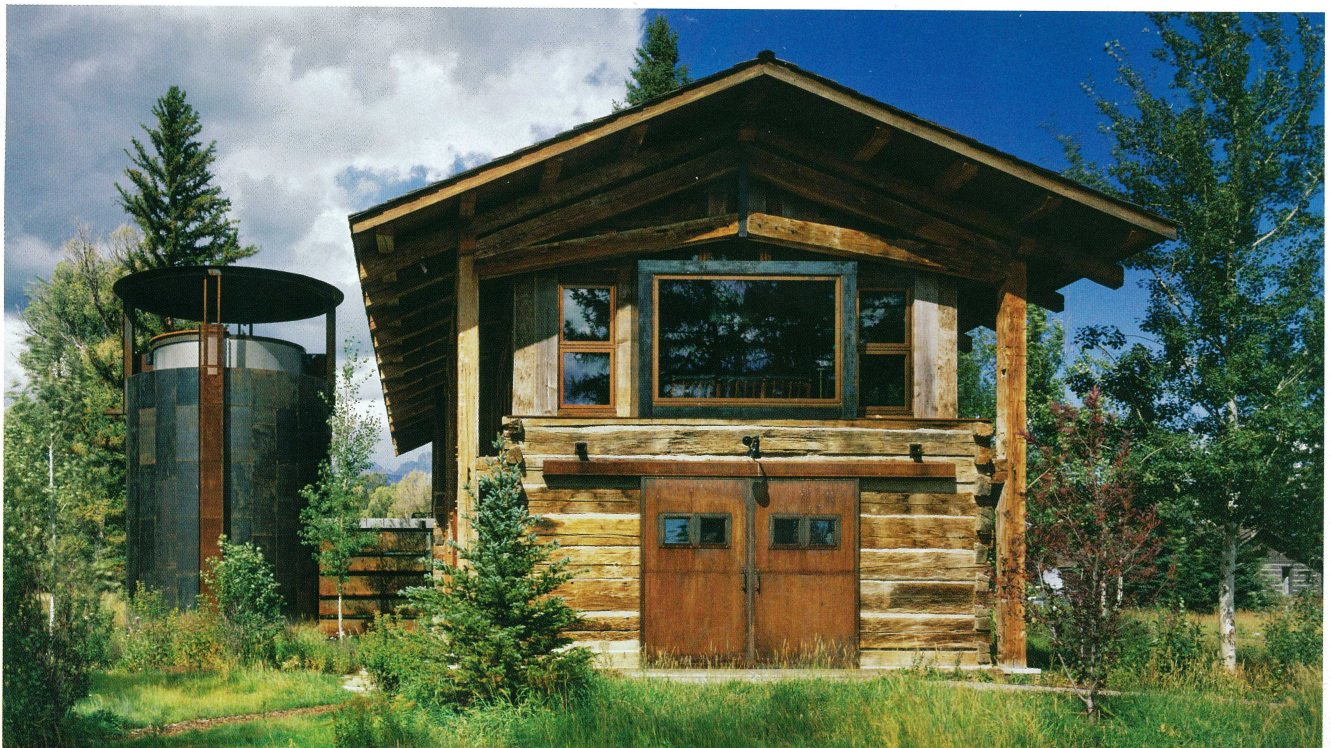
Above: Its most-written-about building may be the Laurance S. Rockefeller Preserve Interpretative Center in Grand Teton National Park. Opened in 2007, it was the first LEED platinum building in Wyoming and the National Park Service. Below: Constructed as a part of a larger residential compound, the Queens Lane Shop Building and Wine Silo makes use of vernacular forms rendered in reclaimed wood and oxidized steel panels.
