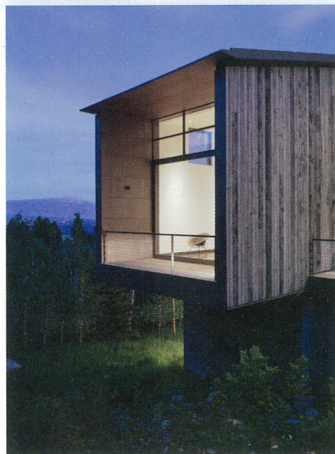
ABOVE: A dramatic view into the kitchen and main living space from the deck. BELOW: Reclaimed wood siding, which was removed from old barns located in the region, requires no finishing or staining.
